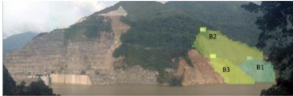
Figura 56 Taludes “B1”, “B2” Y “B3”
